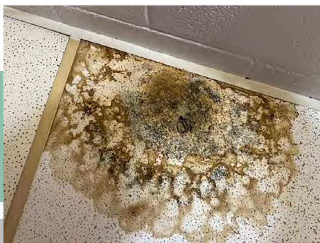
(Top) Mold grows on a ceiling tile in a Richmond, Va., pre-school. (Bottom) In schools without air conditioning, fans do little to keep students cool.
